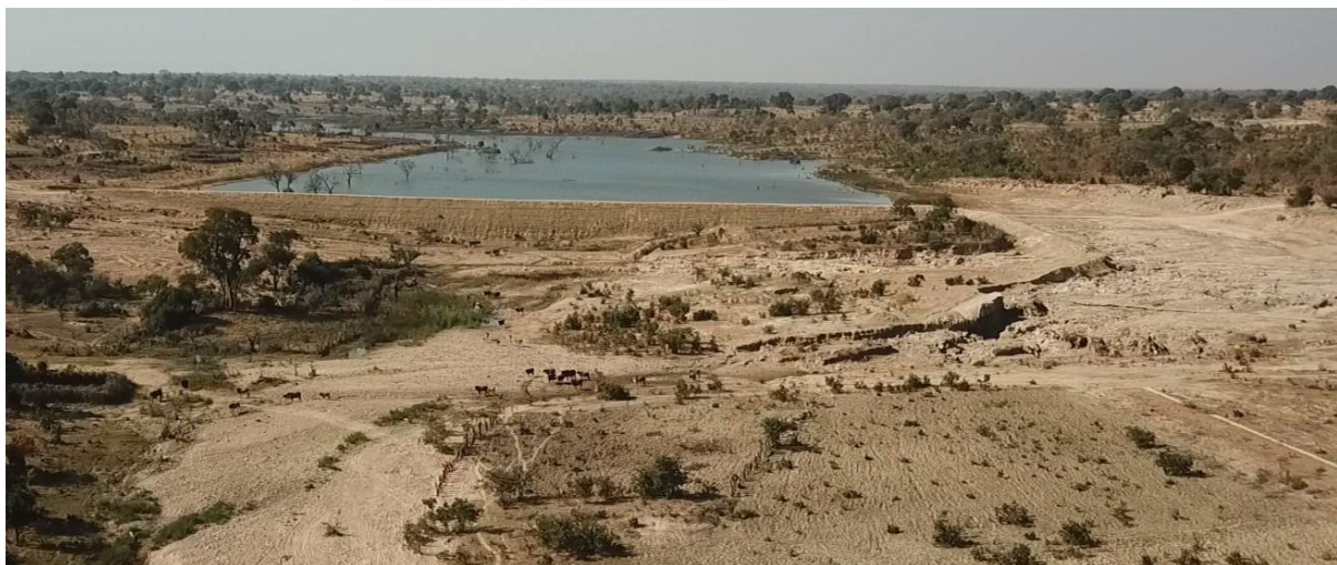
Figure 2: A rehabilitated dam under IDSP (Ngolongozya, Zimba District, Southern Province)
